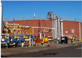
The sludge digesters deal with two streams of 'solids' – sludge from the primary tanks and waste sludge from the reactor/clarifiers (secondary sludge).
