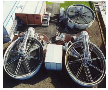
Processing (thickening the solid waste from the reactor/clarifiers) - the DAF system.
