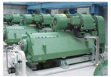
Centrifuges in the dewatering plant complex.
