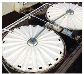
The two gravity thickeners along with the gravity belt thickeners, thicken primary sludge from one and a half percent to three percent solids prior to anaerobic digestion.
