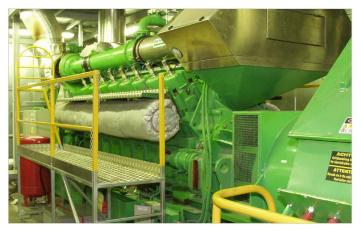
One of the four Jenbacher JMS 616 turbo-charged gas engine/generators.
